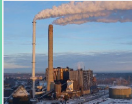
Figure 35: CHP plants in Oulu, Toppila. 185 MW electricity, 320 MW district heat. Fuels peat and wood.
